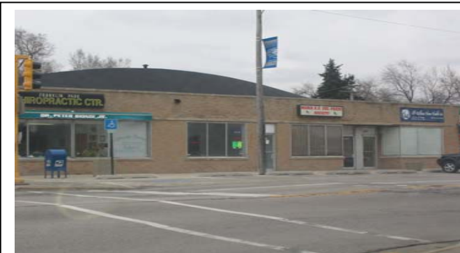
Some commercial structures, like this one-story brick building, could be enhanced by hanging planters, or by relatively minor façade improvements such as additional awnings.
